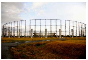
This 137' tall, 1200' diameter "elephant cage" is at Misawa AFB, Japan, for a little while longer. It will be dismantled in 2013, fifty years after its erection, leaving just one operational—near Anchorage, AK.
